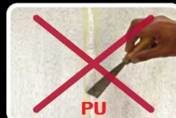
Difficult to tool (PU Sealant)
