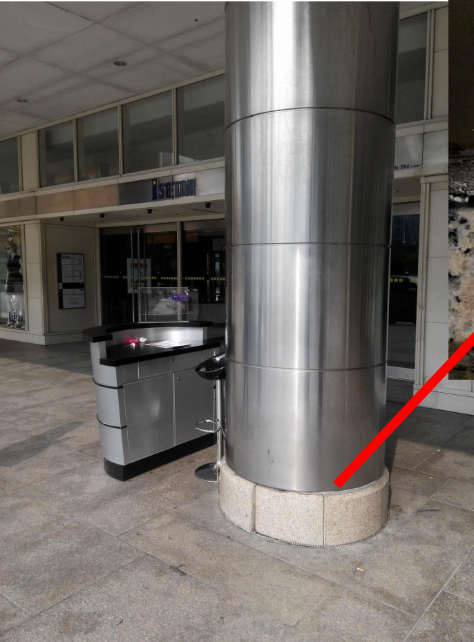
Sealant crazed badly and lost functionality
